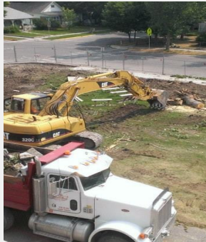
NEW CONSTRUCTION BEGINS AT BROADWATER SCHOOL - SUMMER OF 2014!
